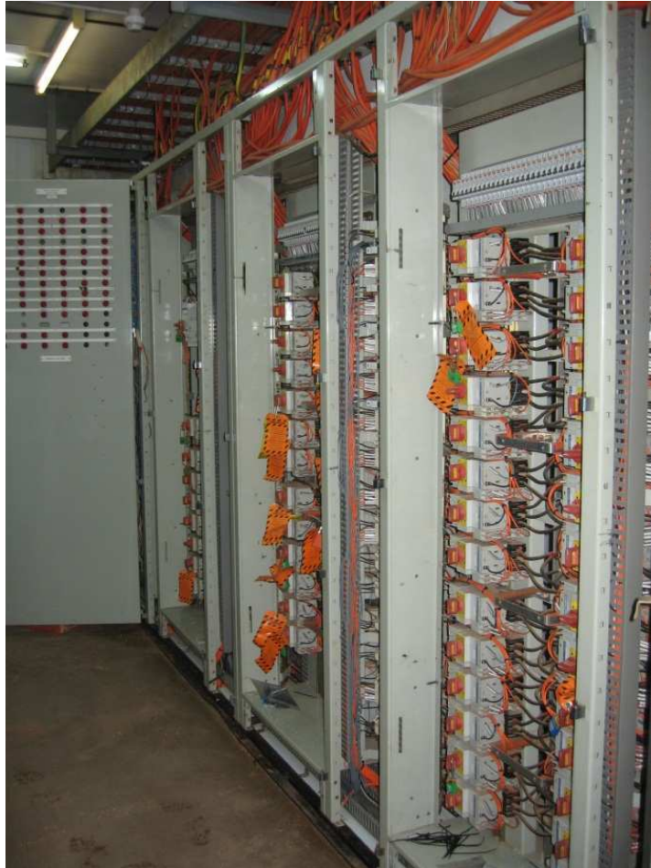
Figure 5: New control wiring installation
