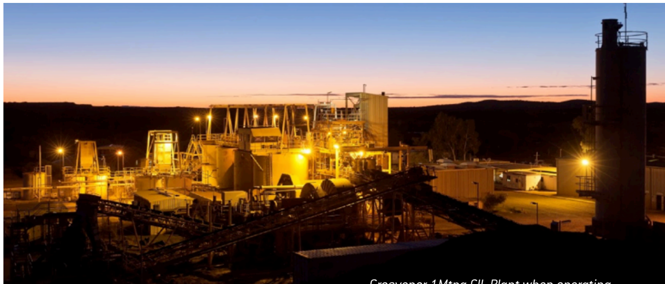
Grosvenor 1.0 Mtpa CIL Plant when operating
